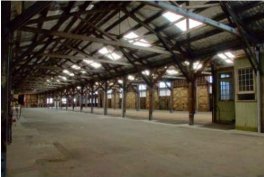
Wooden poles and beams
