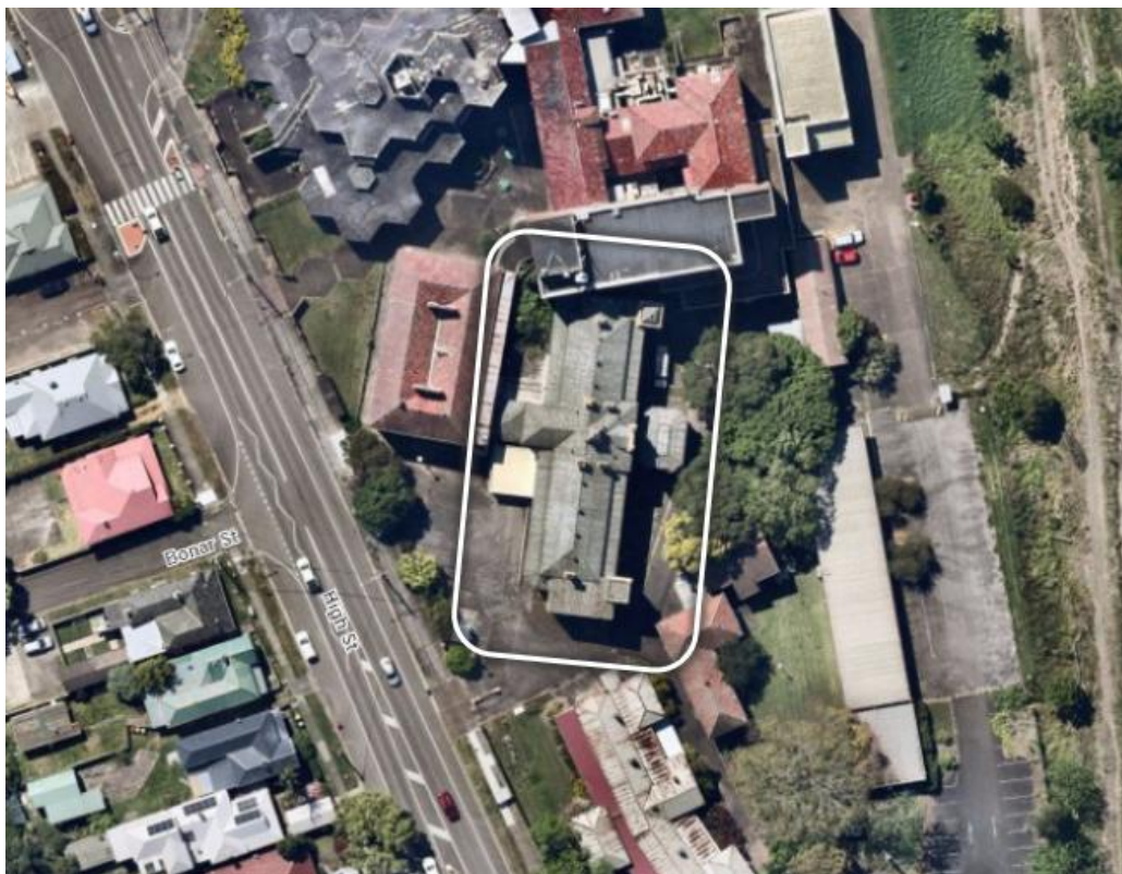
Figure 2: Block J Building
