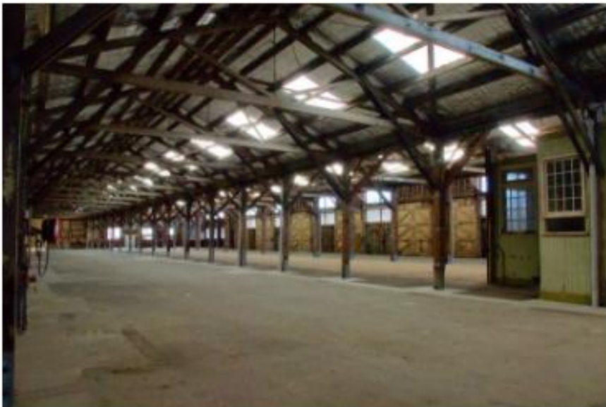
Wooden poles and beams
