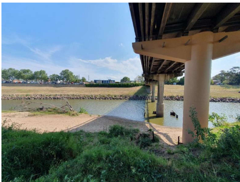
Figure 4-2 Bank erosion under Belmore Bridge
